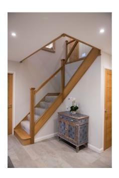
This photo shows the external string clad which has been completed with oak and oak veneer.
