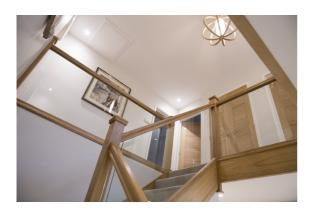
The apron is the section of external string clad which runs horizontally under the landing balustrade.
