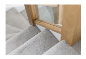
This photo shows an internal string without cladding, the customer has painted it white. The oak below the glass is the baserail which is part of the standard renovation.
